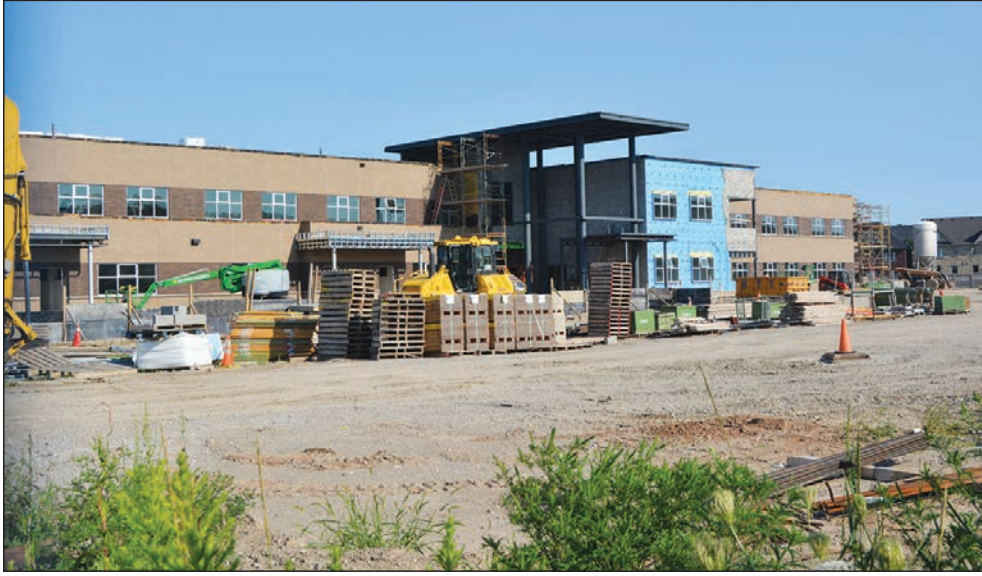
WELCOMING STUDENTS – Tottenham will see two new schools open. Our Lady of Peace Catholic Elementary School on Martin Trail is scheduled to open in November this year. A public school on McGahey Street is now under construction. BRIAN LOCKHART PHOTO
