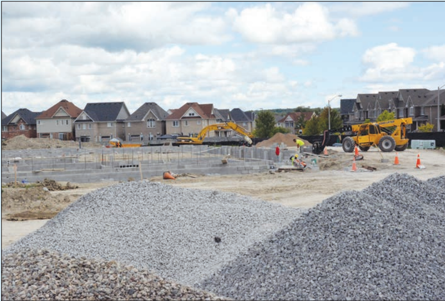
NEW SCHOOL CONSTRUCTION – The new public elementary school in Tottenham is progressing on time, with the land cleared and foundations being laid. The as-yet unnamed public school will be located on McGahey Street. The new school will provide 426 new elementary school pupil spaces. BRIAN LOCKHART PHOTO
